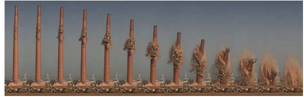
Figure 1. Demolition of a chimney [13].
