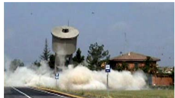
Figure 4. Demolition of a water tower [15].
