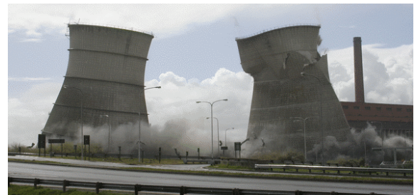
Figure 2. Demolition of the cooling towers [13].
