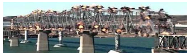
Figure 3. Demolition of a steel bridge [14].
