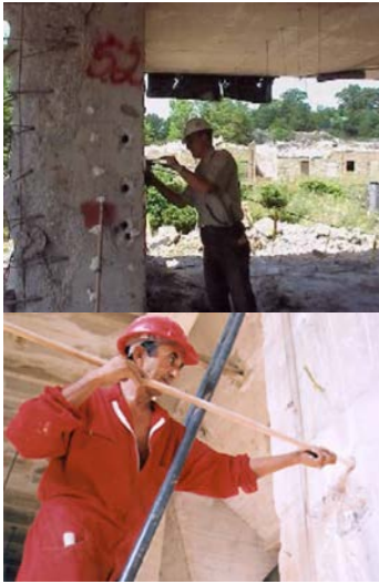
Figure 5. Opening of explosive holes and placing explosives [16].
