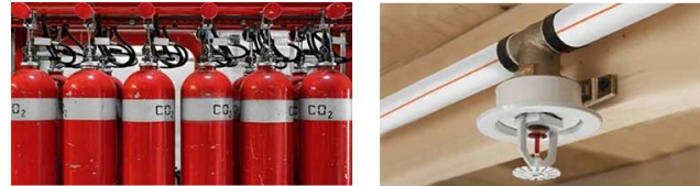
Figure 11. Carbon Dioxide Extinguishing System and Sprinkler Extinguishing System
