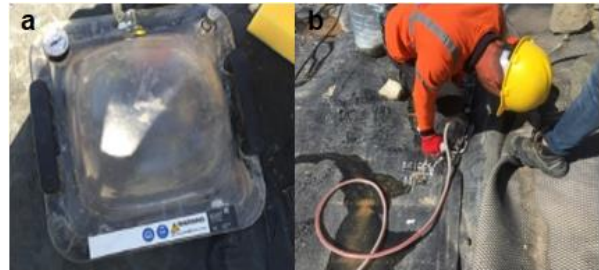
Figure 11. a) Vacuum box [20], b) Vacuum test application.
