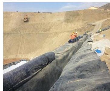
Figure 8. Anchor trench [19].
